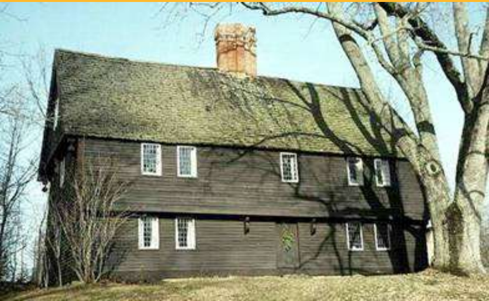
Parson Capen House (1683, Topsfield MA EUA)
